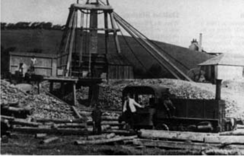
'A Neilson 0-4-0T at one of the iron ore mines worked by Furness Mining Co., possibly Park in 1880.' Kirkman & van Zeller, p. 54.
